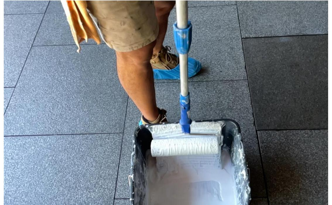
Make sure to soak the roller with sufficient material. See next slide for application procedure.
