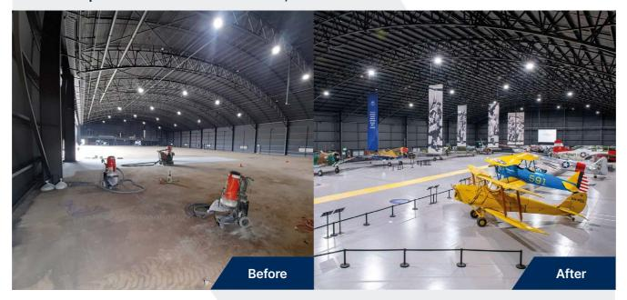
Coating system applied: Luxafloor® LGE and Luxafloor® PTX
